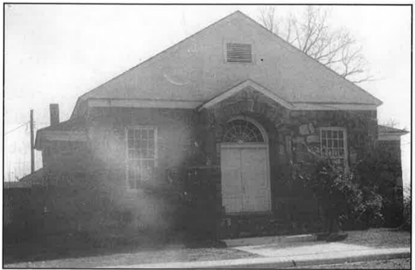
First Presbyterian Church in Jacksonville in its completed state located on Oak Street and South Road.
